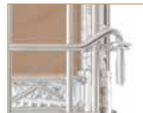
Protective cover on exposed wire ends.
